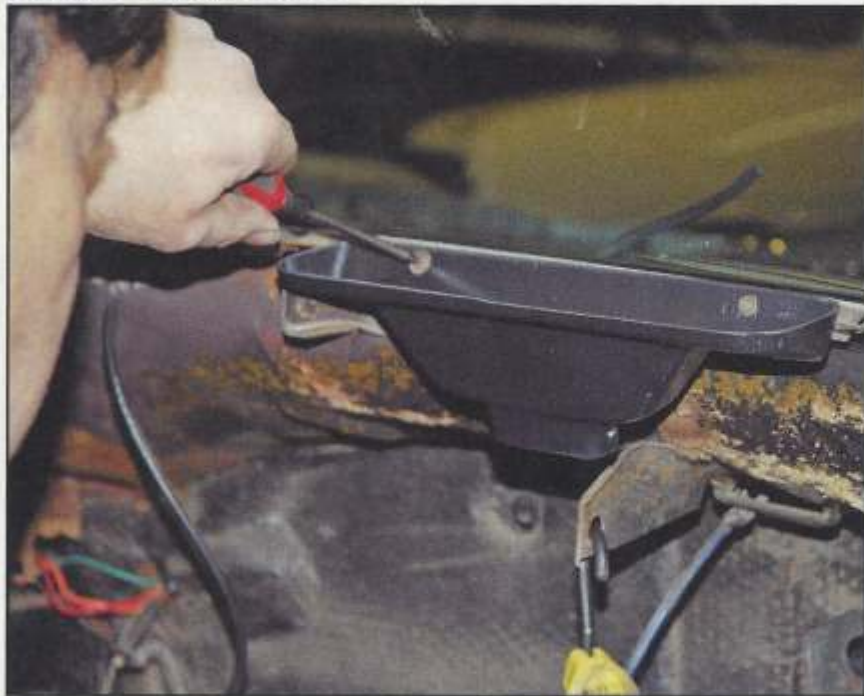
• New defroster ducts are also provided in the kit, and are easily screwed in place once the originals are removed.
