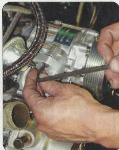
Then the air conditioning compressor is bolted up and the hard lines are installed.
