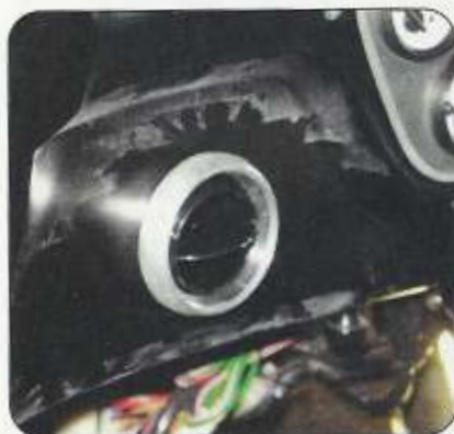
The vents just basically snap into the dash and have little ears that lock them into place. They are very simple to install and they look great in this truck.
