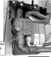
Wrap #10 A/C hose fitting separately with press tape
